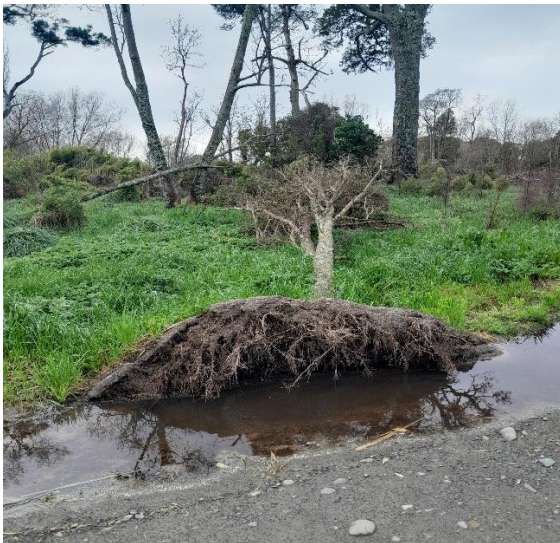
Area one central area cleared of willows and ready to be prepped for planting March 2023
