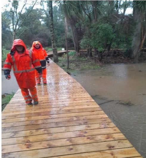
New west side board walk almost completed
